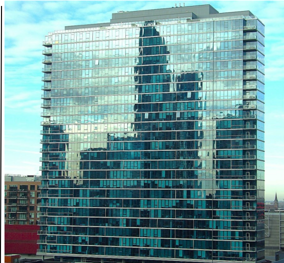
1000 S Clark building reflecting the skyline facing east including the tallest, Helmet Jahn 1000M on south Michigan Ave.
