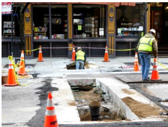
Essential workers putting in new gas lines on Dearborn St. Making hay while the sun shines. Sandmeyer's Books in the background. Photo from 4/9/2020
