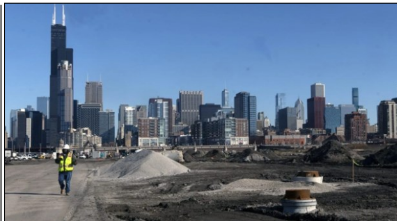
A sole worker walks through "The 78" construction site on March 13, 2020.
