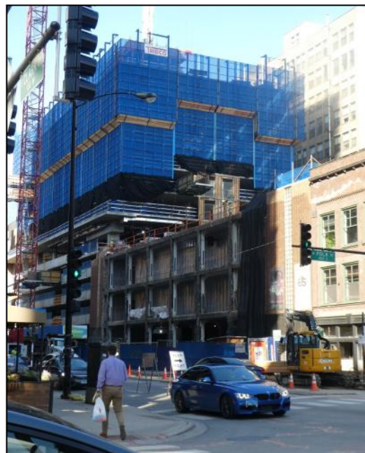
New Apartment building by CMK. Clark near Polk Photo 10/9/2019
