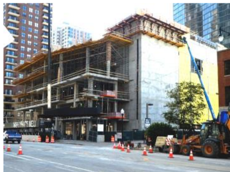
Photo taken Oct 15, 2018. Scheduled completion by the end of 2018. At Wabash and 8th Street.
