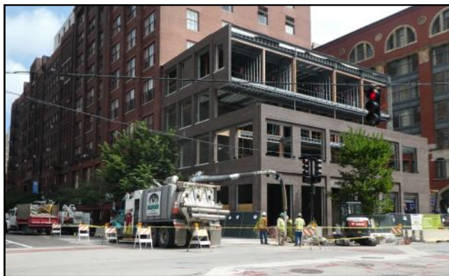
On Thursday, the pedestrian access to Dearborn on the east side of the street was blocked by trucks related to the construction.
