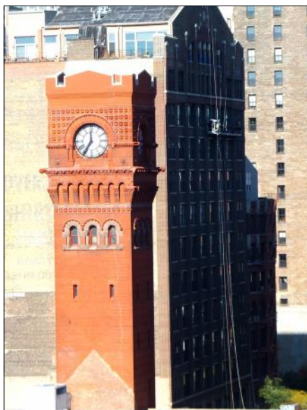
Photo shows façade work being done on the Franklin Building
