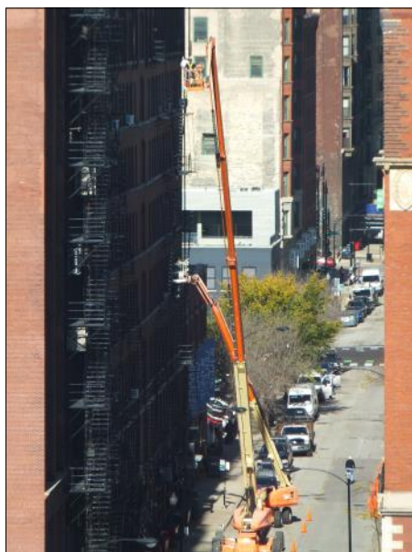
Photo shows window painting work being done on the Donahue Building, Plymouth Ct
