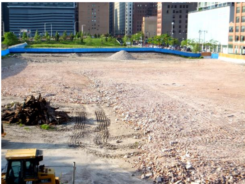
This is the construction site for a planned development just north of River City. Note all the brick that was buried along with railroad ties. This was the location of the old Baltimore and Ohio Train Station.
