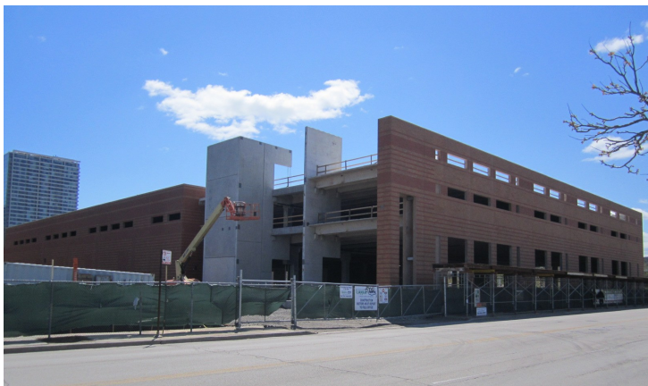
Mariano's with the outside walls up. Expected opening to be in the Fall of 2013. Located on Clark and 17th.
