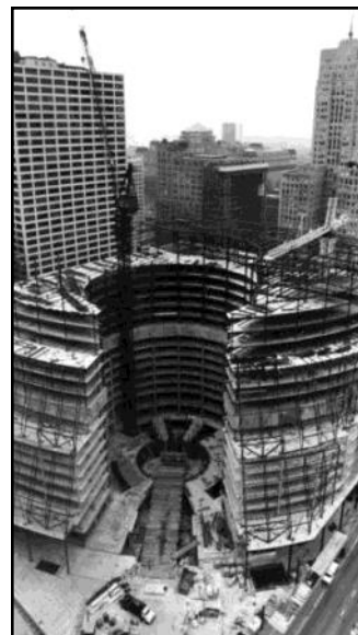
The State of Illinois building under construction in 1982, about the time Paul McGrath got interested in it. Photo/ Chicago Tribune
