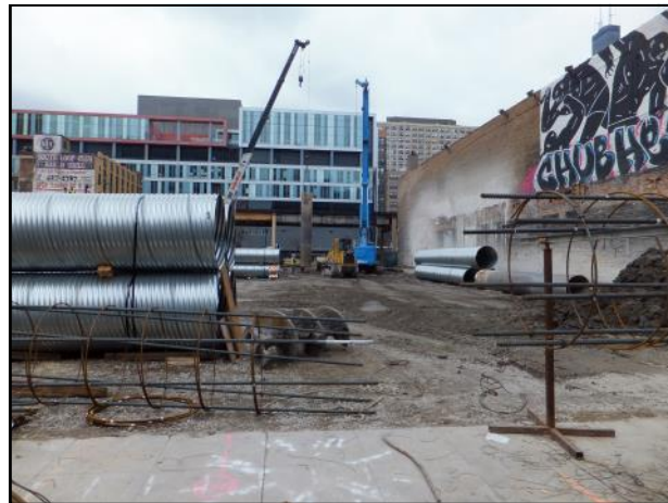
Foundation work has started at the new residence building at Wabash and Balbo.
