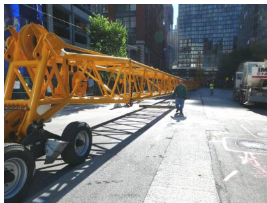
Crane boom stretching from Dearborn to Polk. July 8th, 2018
