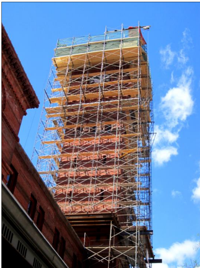
Nip—tuck—point. The historic Dearborn Train Station Tower undergoing restoration.
