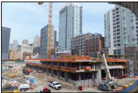
Riverline Project at Wells St and Polk. This is the first of 8 buildings. Progress so far is on the lower garage levels.
