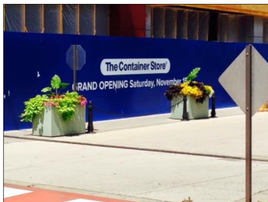
The Container Store Build-out Underway at Roosevelt Collection; Opening November 15th, 2014
