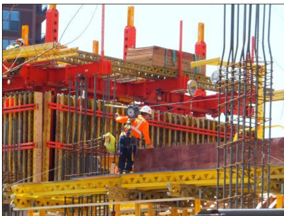
Applying decking on the first level surrounding the elevator shafts on the new apartment building going up at 9th and State.
